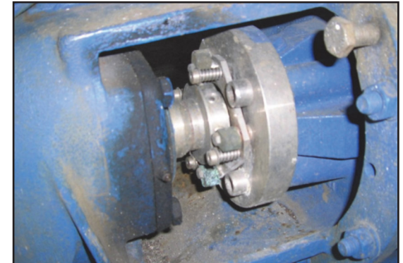
Chesterton 170 Cartridge Slurry Seal installed.
